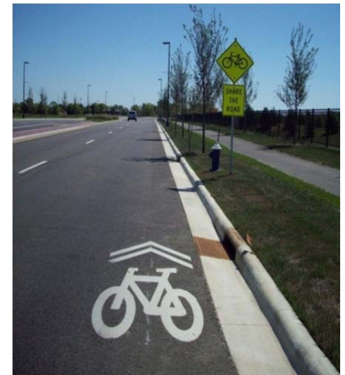
Hilliard, Ohio “sharrow” lane markings and Share the Road signage indicating a shared lane facility.
